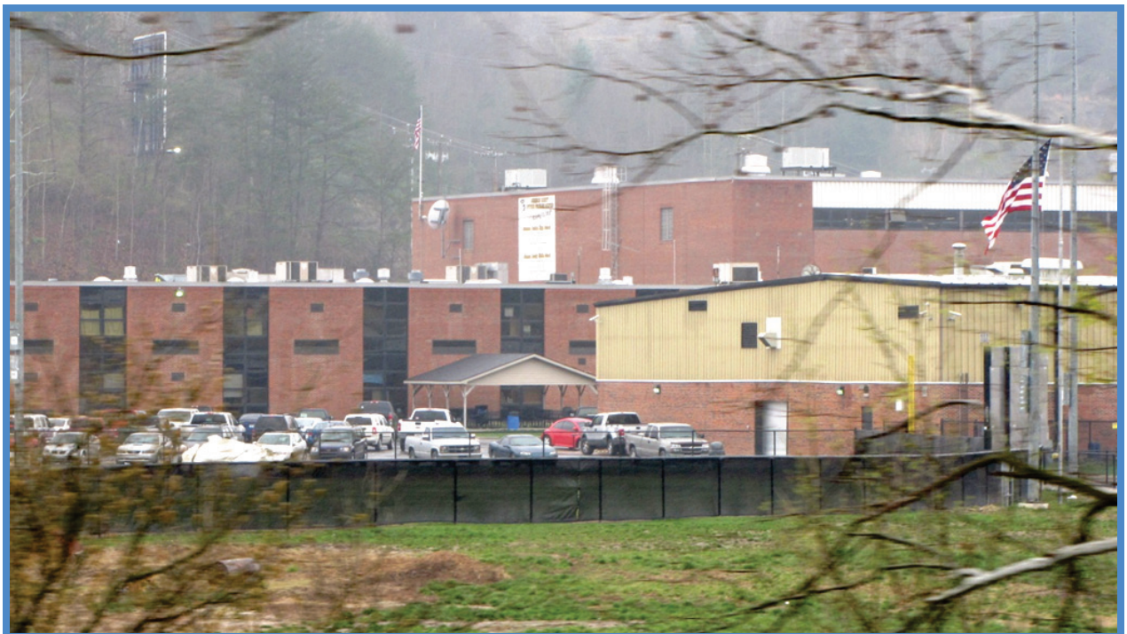
Johnson Central High School and Johnson County Middle School complex
